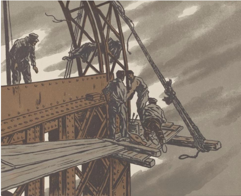
FIG. 4. Riveters at work high on the rising Tower. From H. Rivière, Les trente-six vues de la Tour Eiffel (1902).
